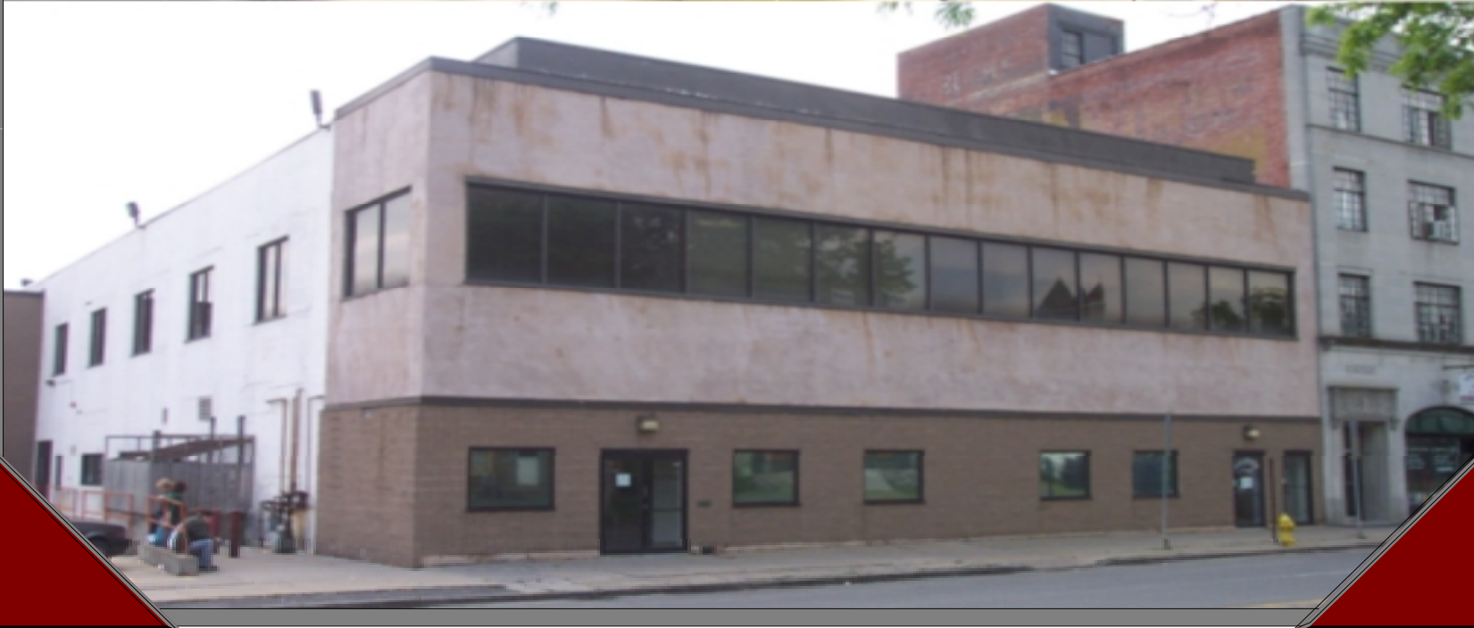
Top: Central New York Services, Inc. Administrative Offices; Bottom: Day Treatment Program Facility
