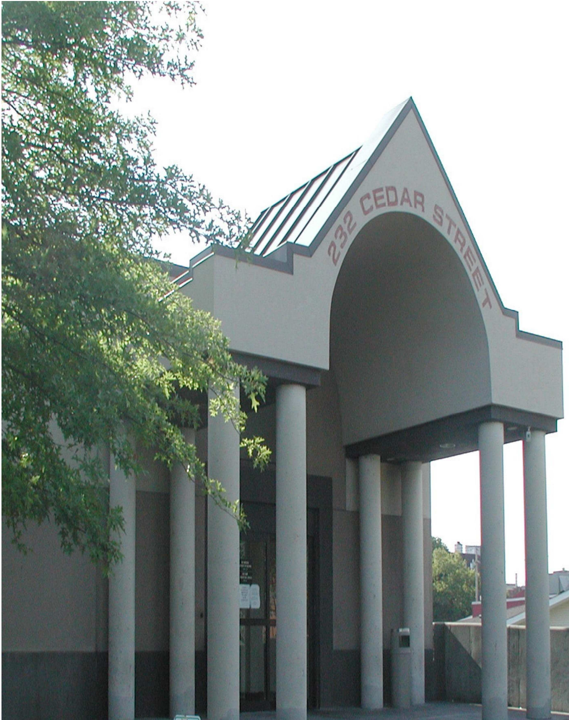
Hill Health Center inpatient detox facility
